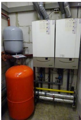
Cv-ketels - warmtapwater
